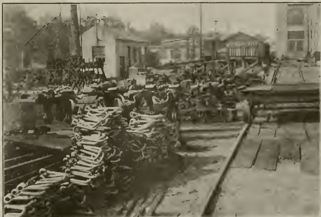
RECLAIMED MATERIAL, RECLAMATION PLANT, VIRGINIAN RAILROAD.
